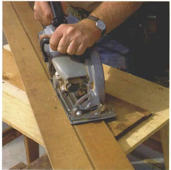
Shooting board for acute angles. A straightedge screwed to a pair of fences guides a circular saw through repetitive cuts that are beyond the swing of the sliding compound saw.
