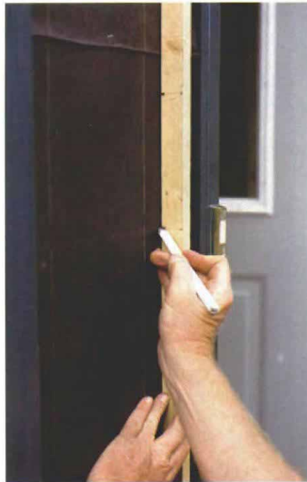
Layout pole. The author uses a water level to locate the bottom courses of siding on all the walls. Then he marks the subsequent courses with the help of a 12-ft. stick with saw kerfs that correspond to the tops of the siding boards.
